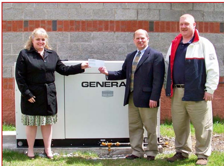
Vicki Myers (left), Friends of Area Agency on Aging Auxiliary President, is shown presenting a check for the purchase and installation of a Generac back-up generator at the Clearfield County Area Agency on Aging’s Meal Production & Distribution Facility. Accepting the check are CCAAA’s Executive Director, John Kordish (center), and Facility and Vehicles Manager, Dave Osterhout (right).
